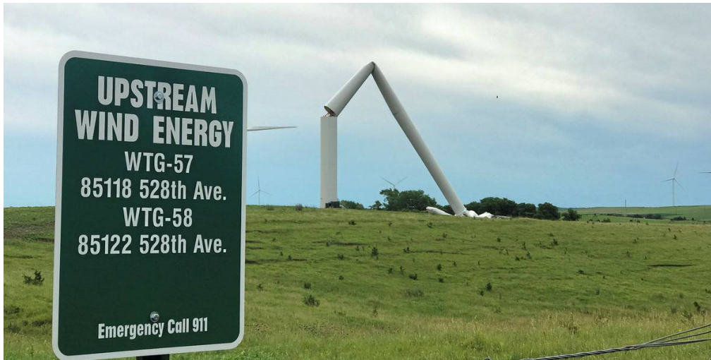
The third in the sequence of turbine collapses in Nebraska. Photo: LuAnn Schindler
